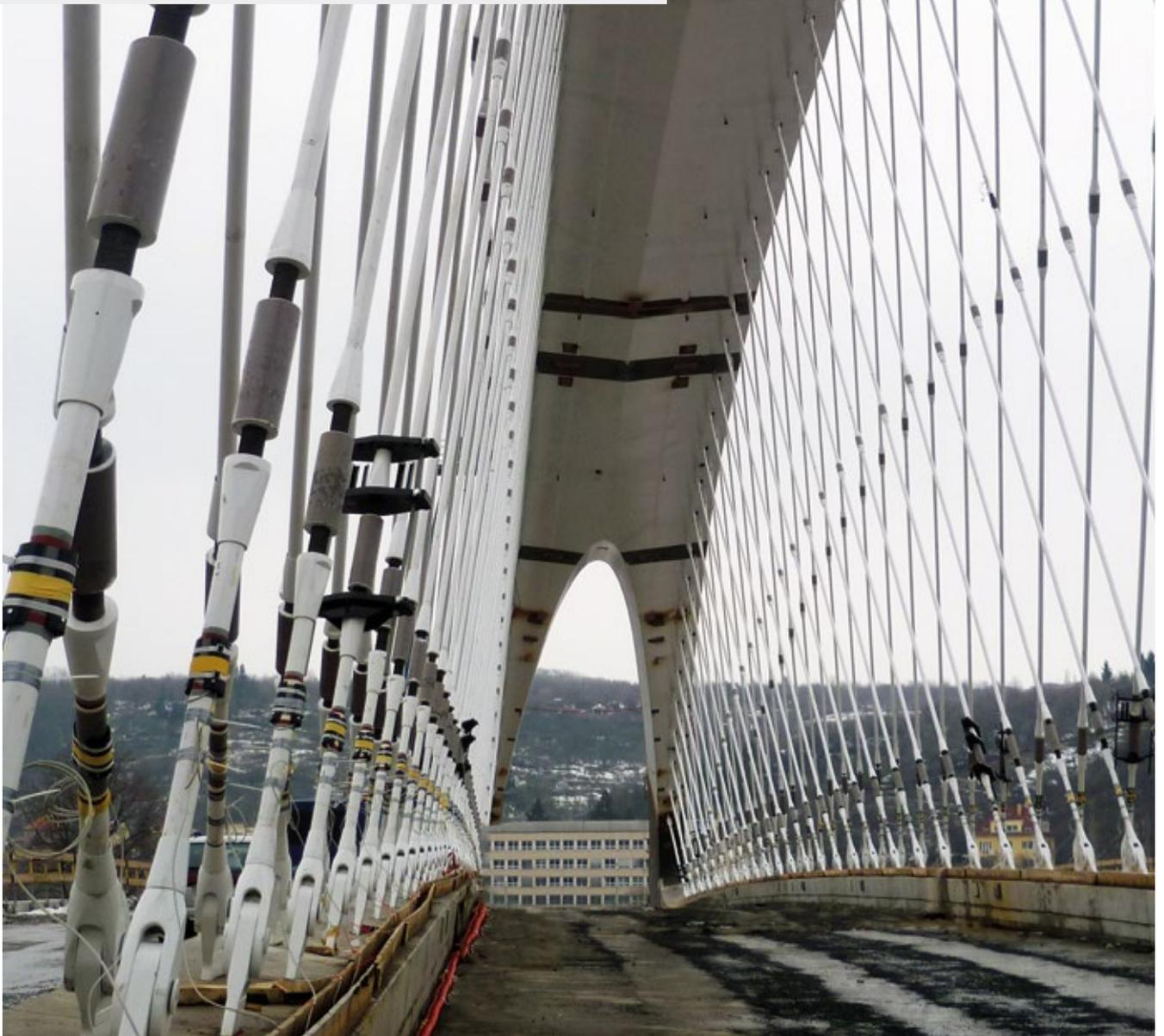
**PONT SCHUMANN** – This two arched stainless steel road and pedestrian bridge in Lyon France opened in 2014 and was designed by Flint and Neil. The carbon steel tendons are designed to support the feature triangular arch sections of stainless steel. The designer required 100% Ex-rays on ALL components, normalised bar material and spherical bearings throughout.
