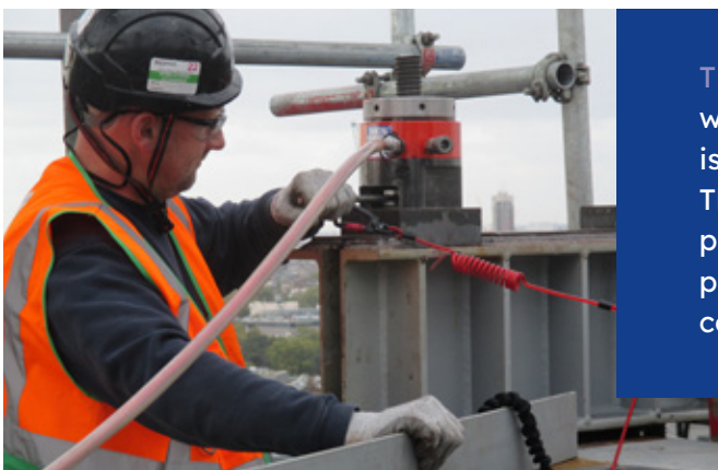
40MM MACALLOY 1030 POST TENSIONING BARS on crane base on Victoria Street, London.
